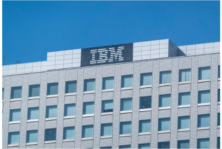
The IBM Hakozaiki Facility building in Tokyo, Japan. Credit: iStock.com/ Marvin Samuel Tolentino Pineda
